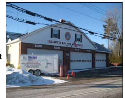
GW Savage/ Water Out of Vermont dries local fire station
