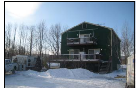
GW Savage/ Water Out of Vermont thaws and dries house in 6 days
