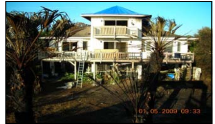
Water Out Northeast Florida dries vacation rental in Tybee Island, GA
