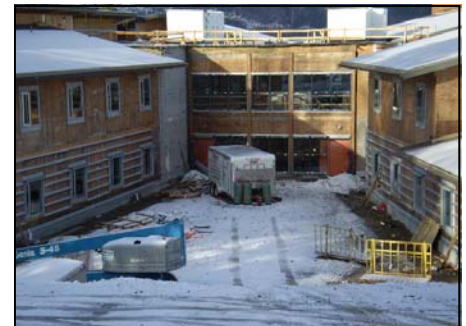
Photos above: Canstar Restoration/Water Out Vancouver dries new construction framing for hospital
