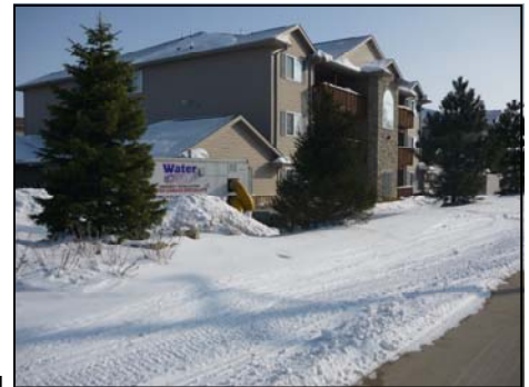
Rainbow International of Quad Cities set up their Water Out trailer to dry condominium in Iowa
