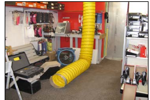
Paul Davis Systems Windsor & Essex dries a two story retail building
